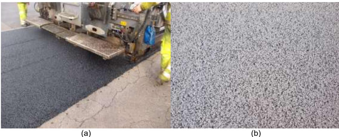
**Figure 3: (a) Paving and (b) the surface of MR6 modified asphalt at Carlisle Airport.**
